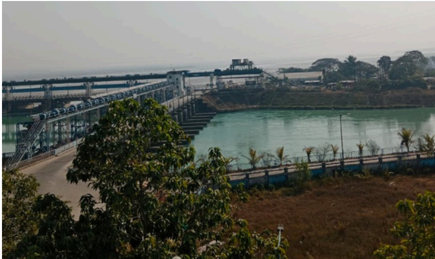
Teesta Barrage and the Canal located in Jalpaiguri District, West Bengal. Sanjit Sakhari
