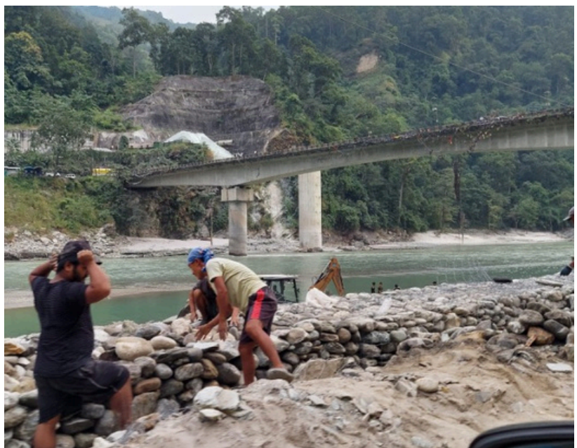
Restoration work near Teesta Bazaar
