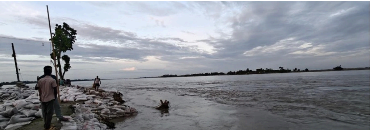
Picture 5: Sandbags stacked along the riverbank to prevent erosion
